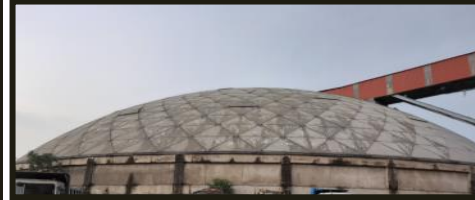
Circular stacker & reclaimer
